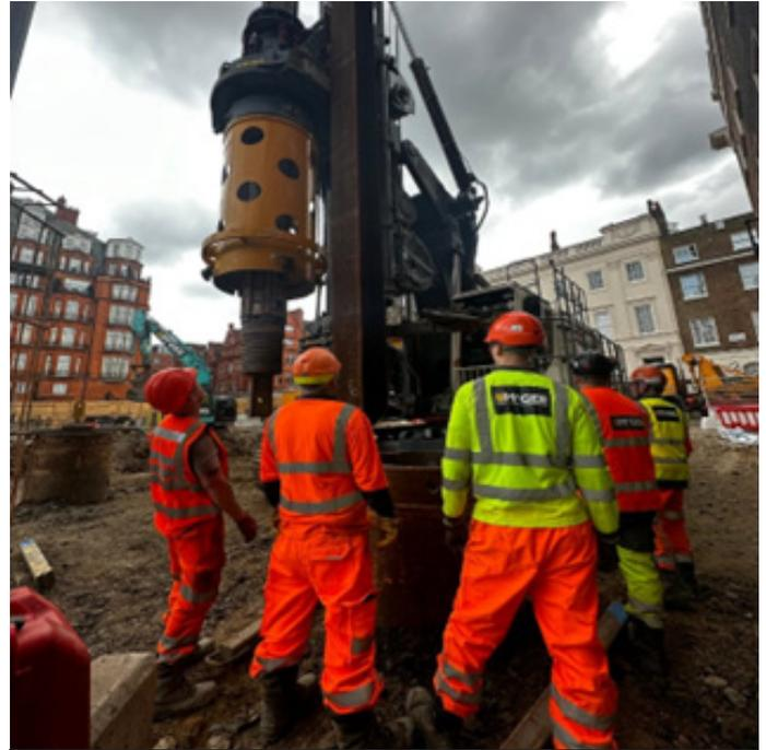
**Plunge column installation for Phase 2 of piling.**
